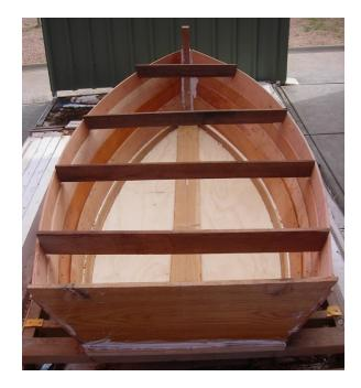
Finally facing the sky; moulds removed and crossspalls inserted to hold the shape while fitting frames, breasthook, quarter and stern knees and thwart (seat). Then removed them all for the next operation!
