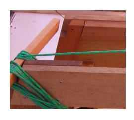
Here is to see the cut in the transom frame which was to accommodate the chine. In this first attempt I laid the chine on top of the transom and projected the chine section down to obtain the cut out. When the chine was cut to length and lowered into the frame it was too short!
